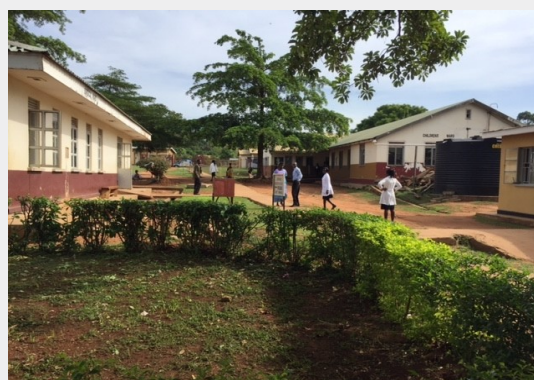
Image of a hospital in Gulu, Uganda
